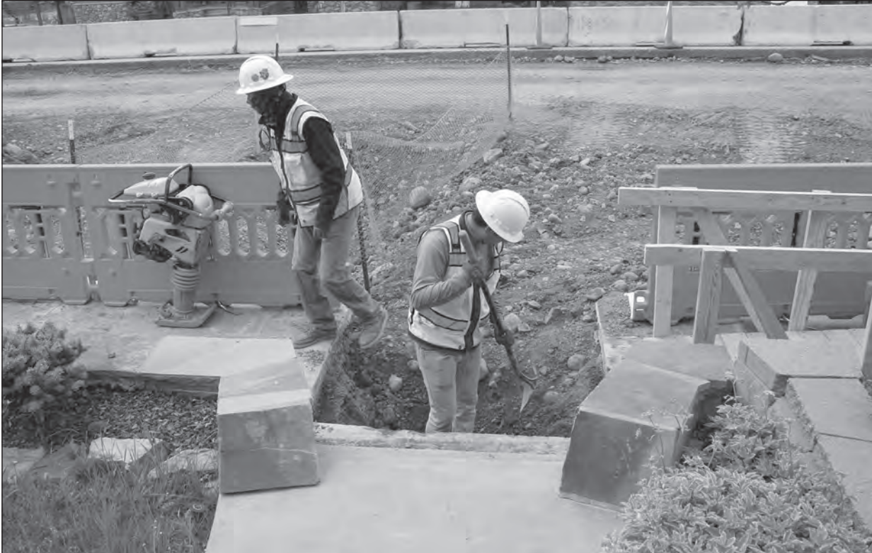
SUN photos/Shari Pierce Construction workers work to fill in a hole following the replacement of a sewer lateral line on Wednesday, May 14. Crews are working to replace water and sewer lines throughout the work zone while maintaining business access.
