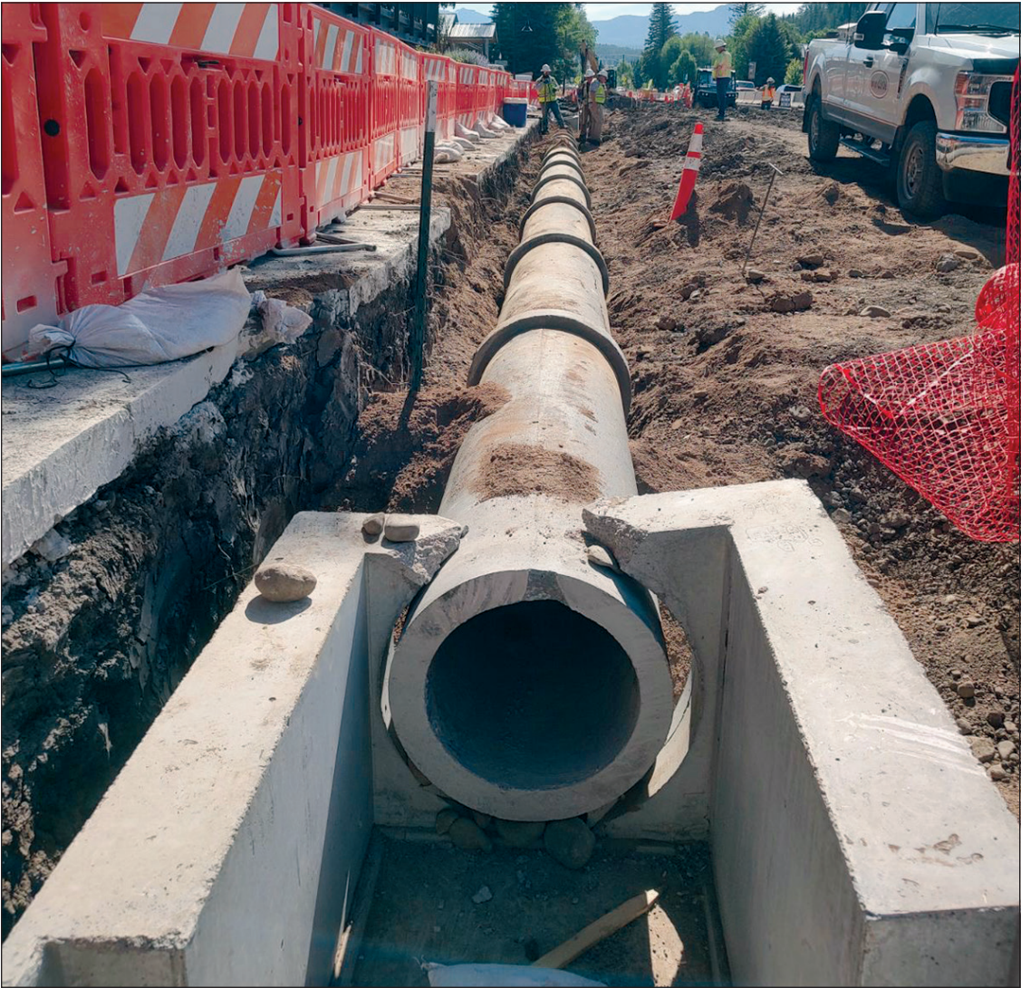
Photo courtesy Colorado Department of Transportation New storm drain installation takes place along U.S. 160, with 110 feet of 18-inch reinforced concrete pipe that connecting the upstream inlet structure to the downstream structure at 2nd Street where it crosses U.S. 160.
