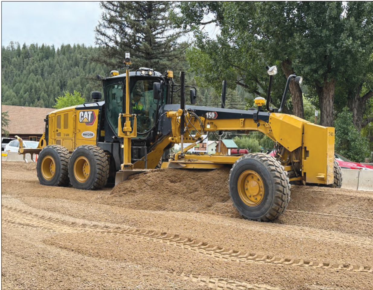
Photo courtesy Colorado Department of Transportation U.S. 160 reconstruction workers grade the aggregate base course between 1st and 3rd streets ahead of concrete paving, which is now slated to begin the night of Thursday, July 31. The second phase of paving on the stretch is planned to take place overnight on Aug. 6.
