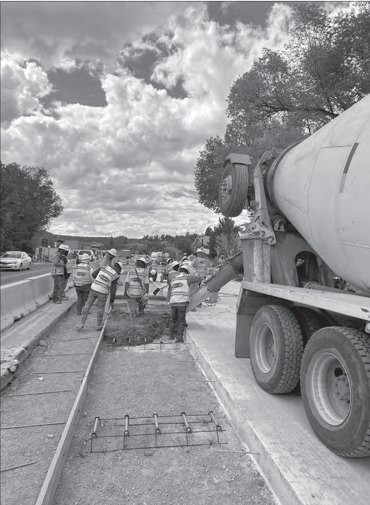
Photo courtesy Colorado Department of Transportation Hand pouring of concrete continues. Once the roadway flat work is completed, crews prepare for curb, gutter and then sidewalks.
