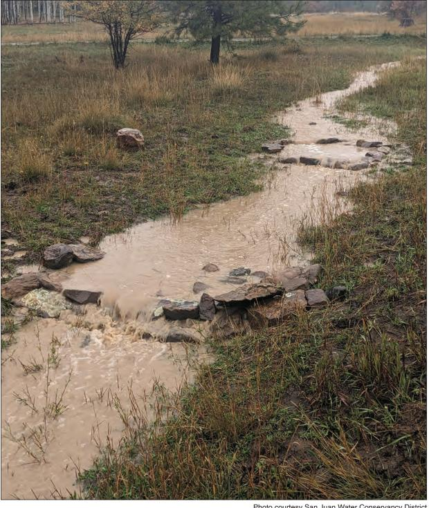
Photo courtesy San Juan Water Conservancy District Watershed restoration structures worked as planned during recent heavy rains.
