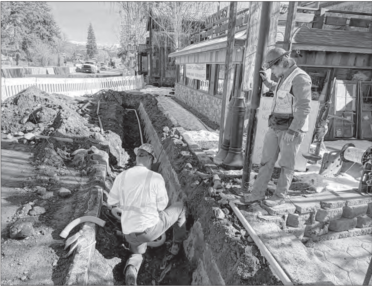
Photo courtesy Colorado Department of Transportation Construction crew members work on stormwater utilities along U.S. 160. The Colorado Department of Transportation notes stormwater utility work requires coordination with multiple utility agencies, such as electric, to mitigate potential conflicts.
