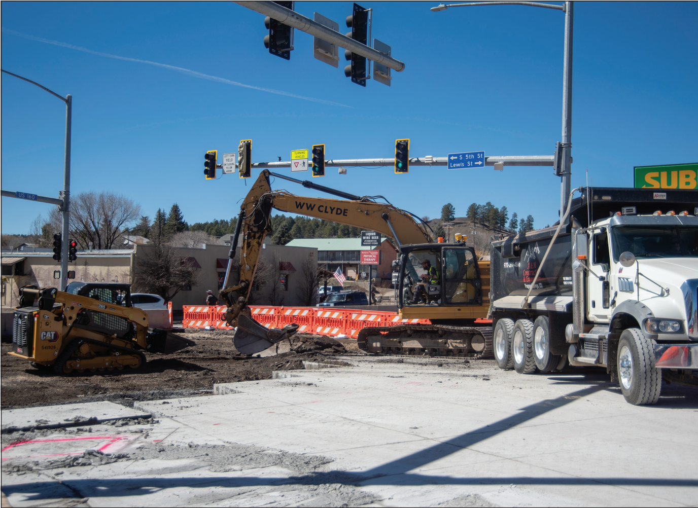
Crews work on removing the old roadway surface at Lewis Street and U.S. 160 on Wednesday, March 18. The underground utility work at the intersection will include demolition and replacement of the geothermal, water and sewer lines before the intersection is built back with ADA-accessible curb and gutter and concrete paving.
