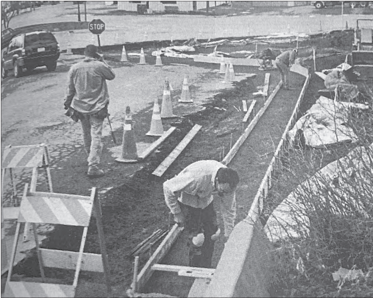
From the March 30, 2000, Pagosa SUN — The revised three-way intersection at U.S. 160 and Lewis and 5th streets is starting to take shape as sub contractors Joel Kostachek (Absolute Rock & Concrete), left, and Danny Gravely (ABC Construction), foreground, align the forms for new curving and gutters Wednesday morning.
