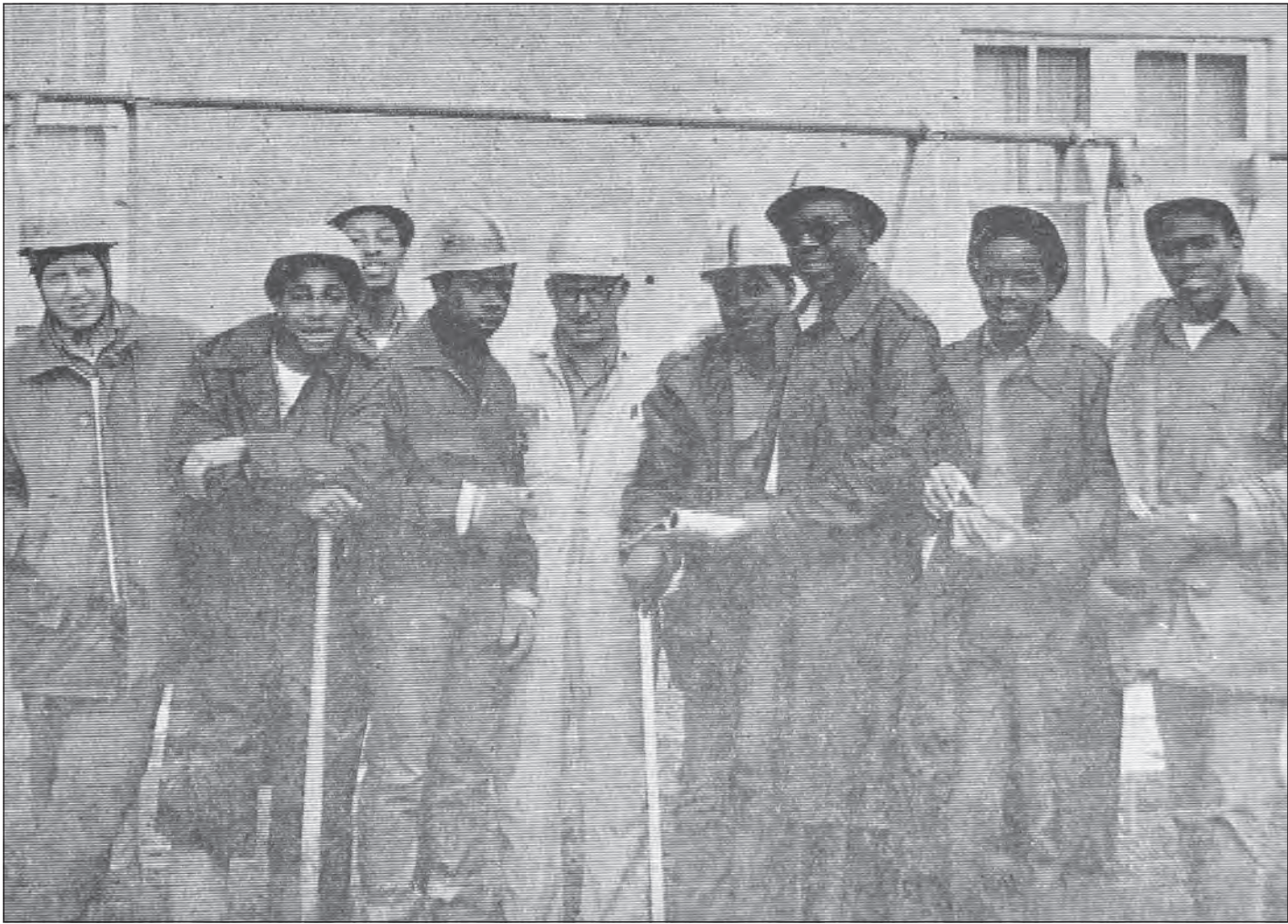
From the April 18, 1968, Pagosa SUN — HEAD START HELP – This group of Job Corpsmen, under the direction of Henry Snow (light coveralls) installed playground equipment for children in the Head Start program. The equipment was installed just north of the Parish Hall the first of the week where it will be convenient for the children. This is one of the many public service projects performed around the community by the Job Corps.
