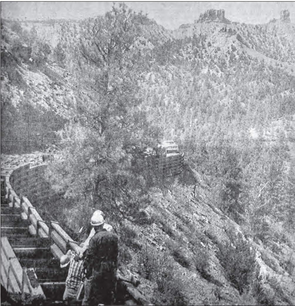
From the April 30, 1970, Pagosa SUN — NEW ROAD — A new road, being constructed to the Chimney Rock Archeological Area by the Forest Service, has an easy grade and is being held on the side of the mesa by bins. The large chimneys of Chimney Rock are visible in the background. The new road will terminate a few hundred yards from the chimneys.
