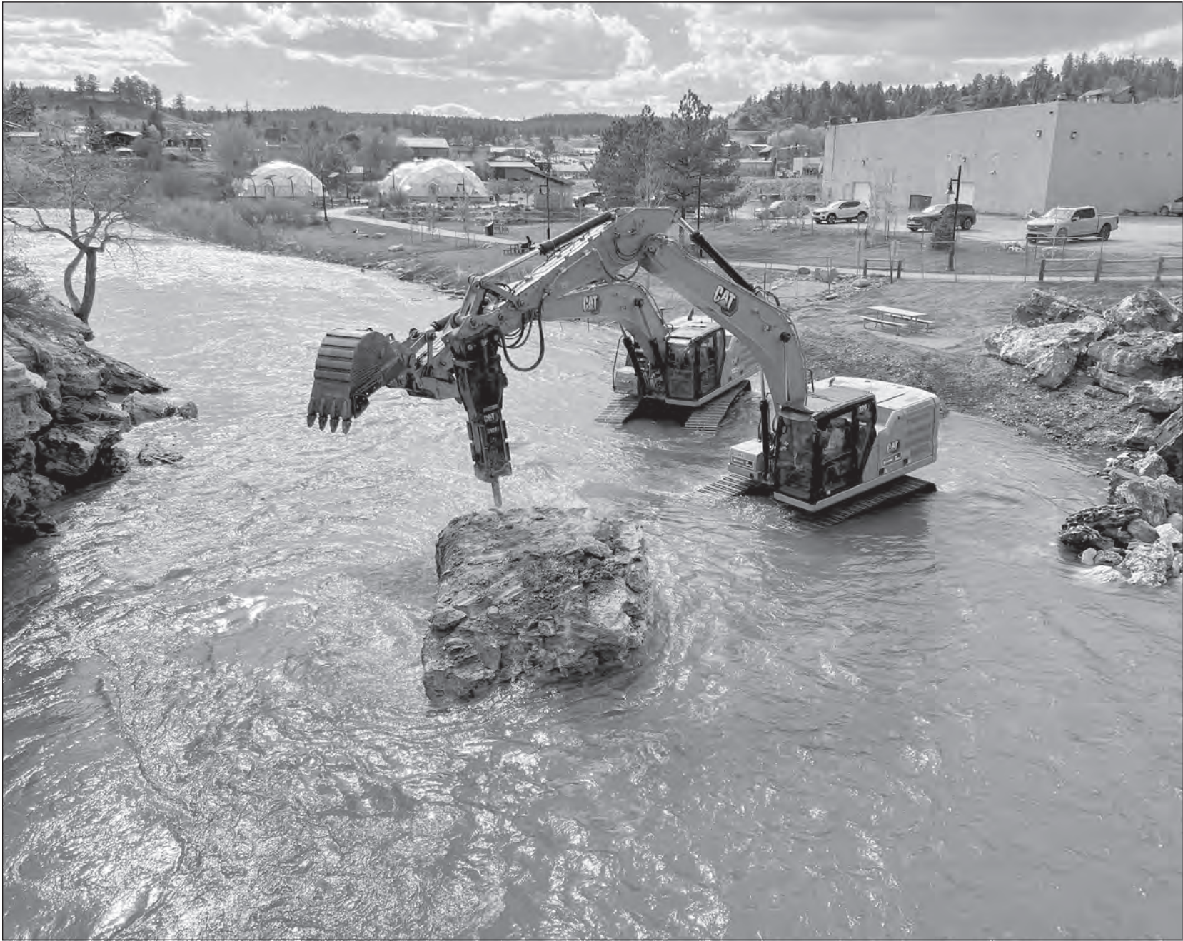
SUN photo/Shari Pierce Post-flooding work continues in the San Juan River near Centennial Park on Friday, May 8. Work included crushing large travertine boulders for bank stabilization.
