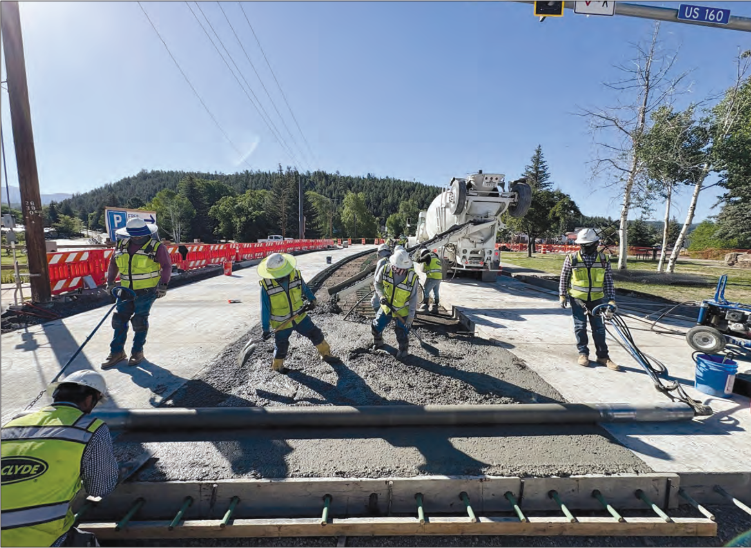
U.S. 160 reconstruction personnel work to pave the Hot Springs Boulevard intersection. Paving operations at the intersection are anticipated to be completed by the end of the day on Thursday, June 18, allowing for the reopening of Hot Springs Boulevard to traffic, as well as open the overlook parking lot.
