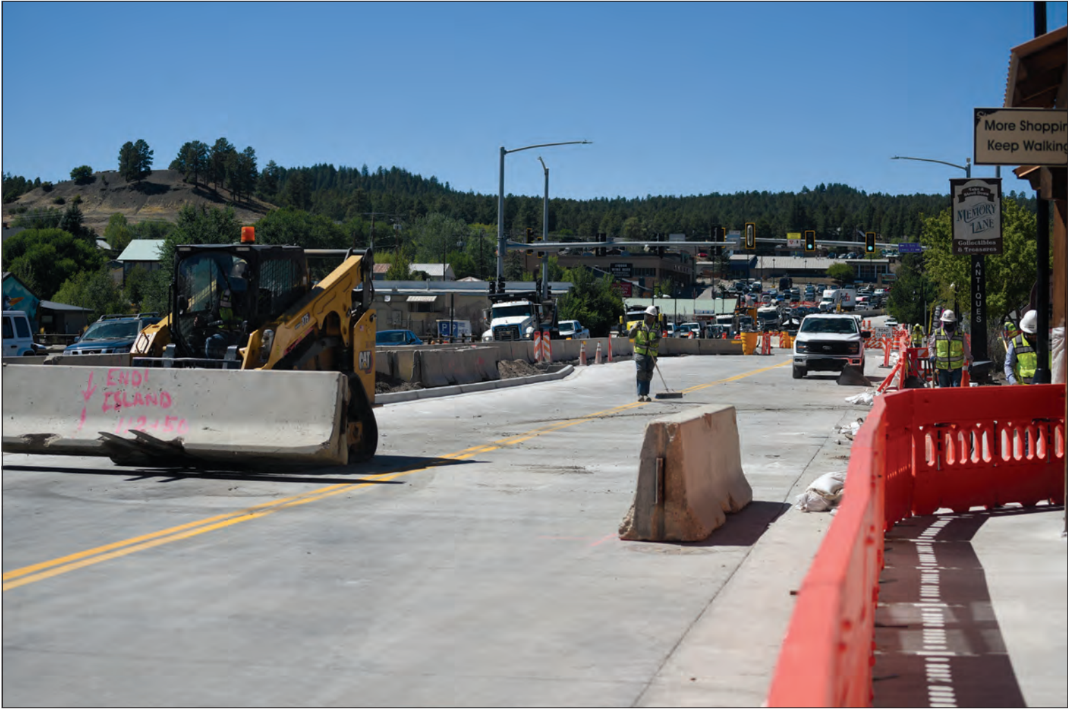
Crews continue work on U.S. 160 in downtown Pagosa Springs ahead of next week’s planned traffic shifts. According to project personnel, there will be multiple traffic shifts in the coming weeks as work continues.
