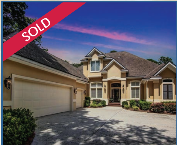
25504 Marsh Landing Parkway Marsh Landing
