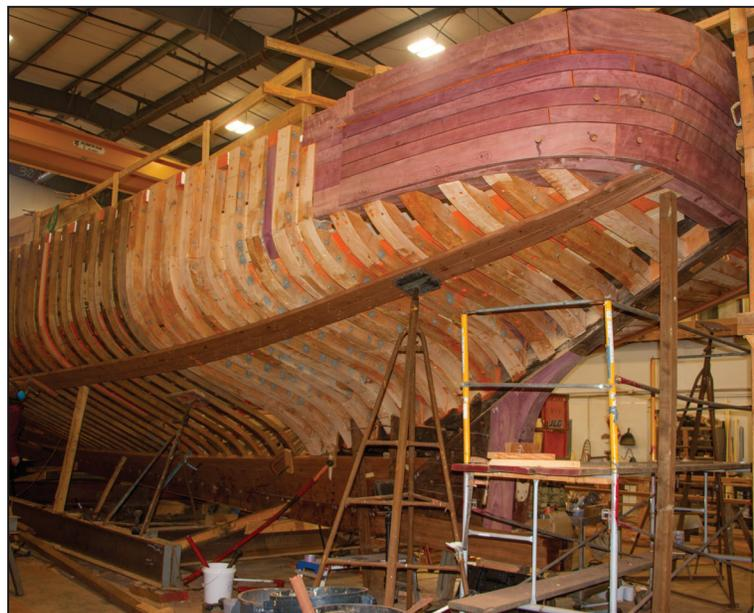
The graceful lines of the Western Flyer are on display in this view of the port flank. Ribs have been bent into place, ready for planking to be laid up, sealing the new hull of the 1937 purse seiner built in Tacoma for the Monterey, California, sardine fleet.
