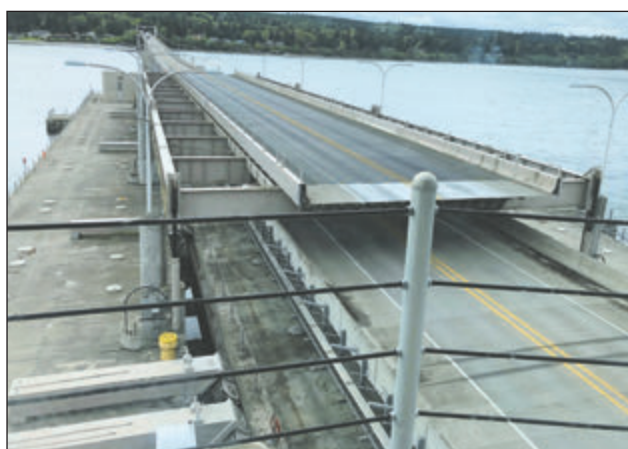
The Hood Canal Bridge during an opening period. Photo courtesy of the Washington State Department of Transportation
