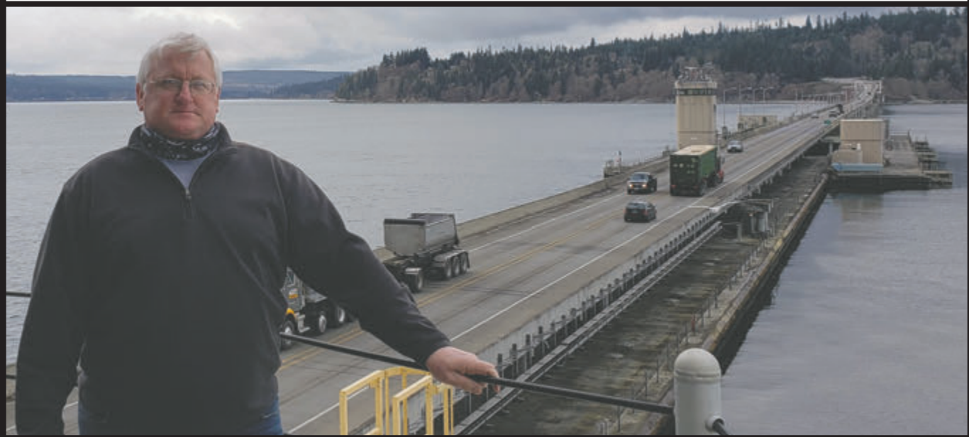
Above, Paul Gahr, who grew up in Port Townsend, is the supervisor for the Hood Canal Bridge.
