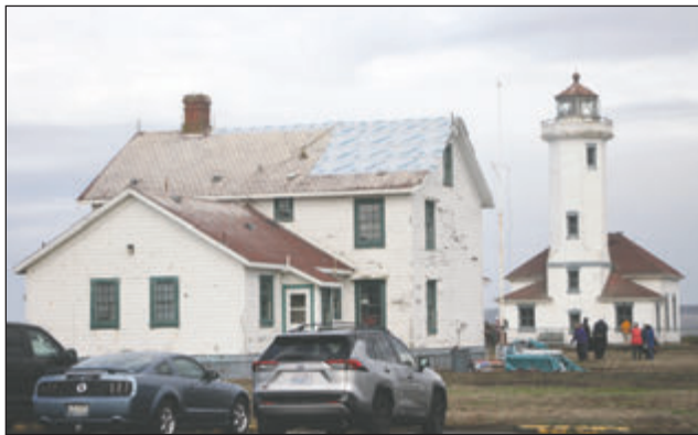
A heavy windstorm on Sept. 17 destroyed part of the keeper's house roof, leaving a large portion of it exposed to the elements. The next stage of the Lighthouse Society's preservation plan will replace the roof of the keeper's house. Leader photo by James Sloan
