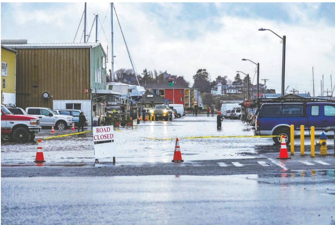
A King Tide and a 9 ft. storm surge in December of 2022 flooded businesses in the Port Townsend Boat Haven Marina.
