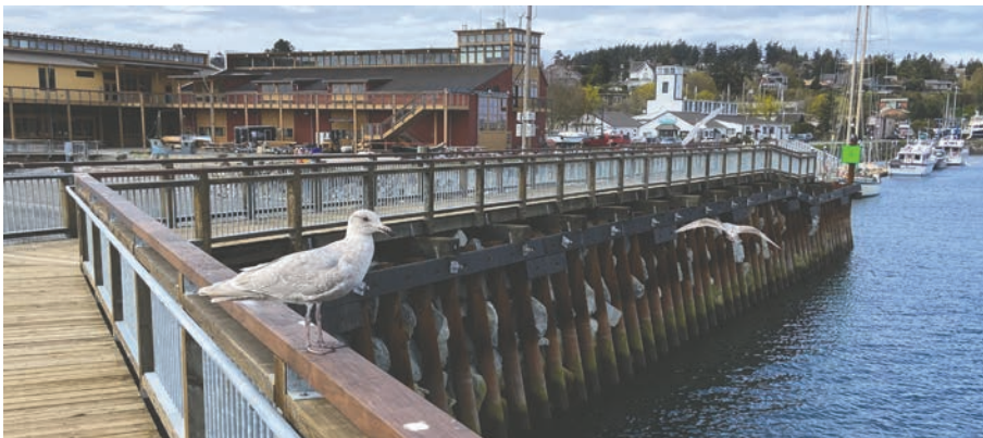
The new jetty walkway is next to the Northwest Maritime Center.
