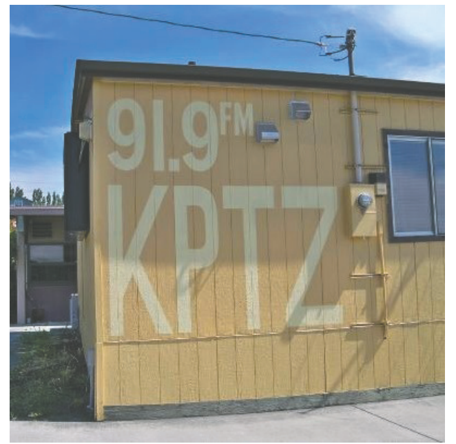
The former KPTZ building at the Mountain View campus will be open to new tenants soon. Leader file photo
