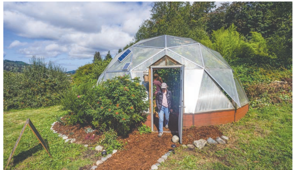
Also at Kodama Farm, a geodesic dome greenhouse is home to species of tropical and sub-tropical plants including lemon, lime, kumquat, blood orange, starfruit, cardamom, banana and passion fruit. It is heated passively through thermal mass and a solar powered "climate battery," a sign outside the greenhouse states. Leader photo by Nicholas Johnson
