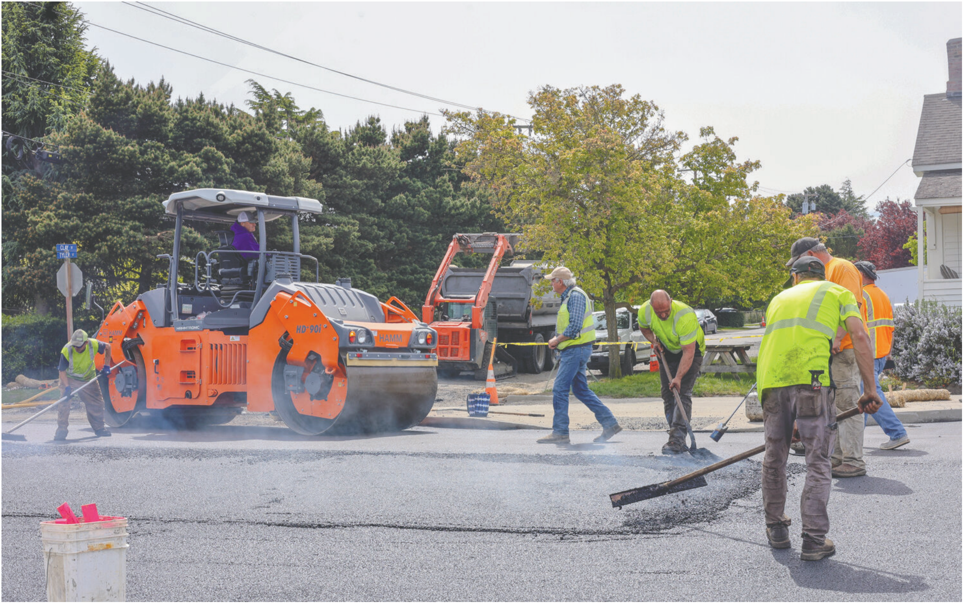
Northern Asphalt crews packing down new asphalt on Tyler Street on May 8. Courtesy photos
