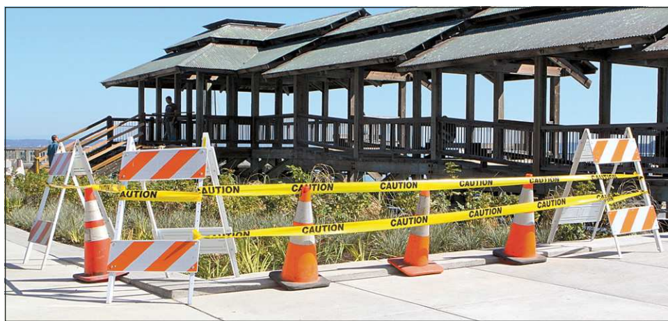
This raised lip on a portion of the new curb next to the waterfront wave gallery has caused at least one sightseer to trip. According to city officials, the problem is to be addressed by installing a bench or railing.
