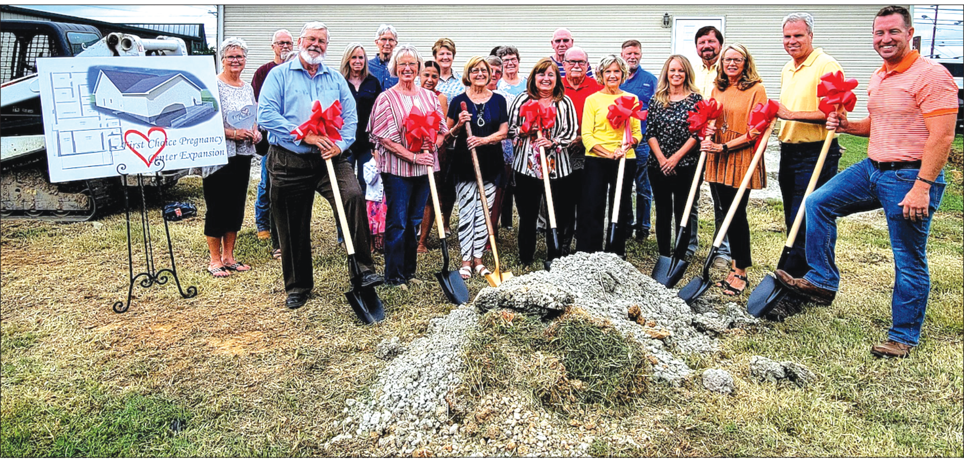
T-G Photo by Zoe Haggard First Choice Pregnancy Counseling Center has been open for 22 years. So there were a lot of smiles by staff recently as the center conducted a groundbreaking for its new addition—one which will help expand the “Baby Boutique.” With shovels ready to move dirt are, from left, John Davis of Davis Stokes Collaborative; Dottie Mershon; Pam Cooper; First Choice Director Angela Rasnick; Bonnie Saunders; Lisa Turner; Steven Flippo, from Hawkins and Price; and Josh Bobo. Other members of the community (back) attended the event also.
