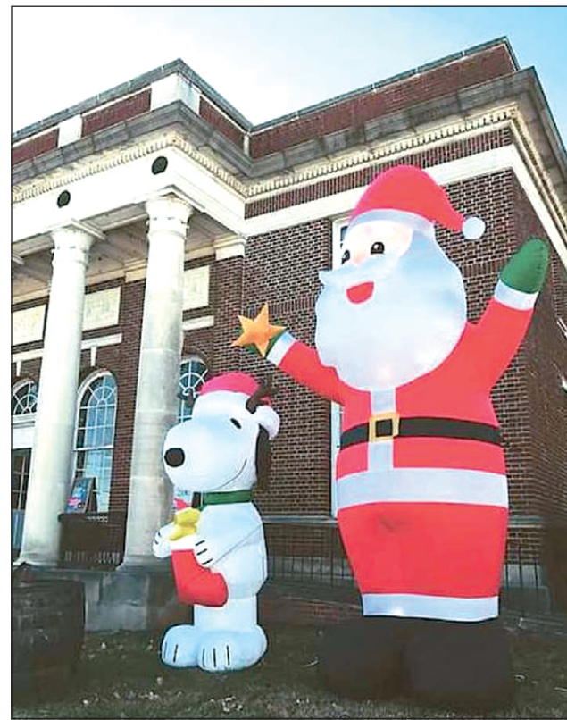
Submitted Photo The Shops at Main & McGrew—located in the former public library on the square—went all out for Black Friday and Saturday's Small Business event. Danielle Armbruster, owner, said despite all the construction, she wanted to give the historic public square a merry Christmas look.
