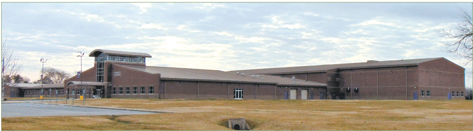
The new west wing of Community High School will be built on the right side (when facing the building).
