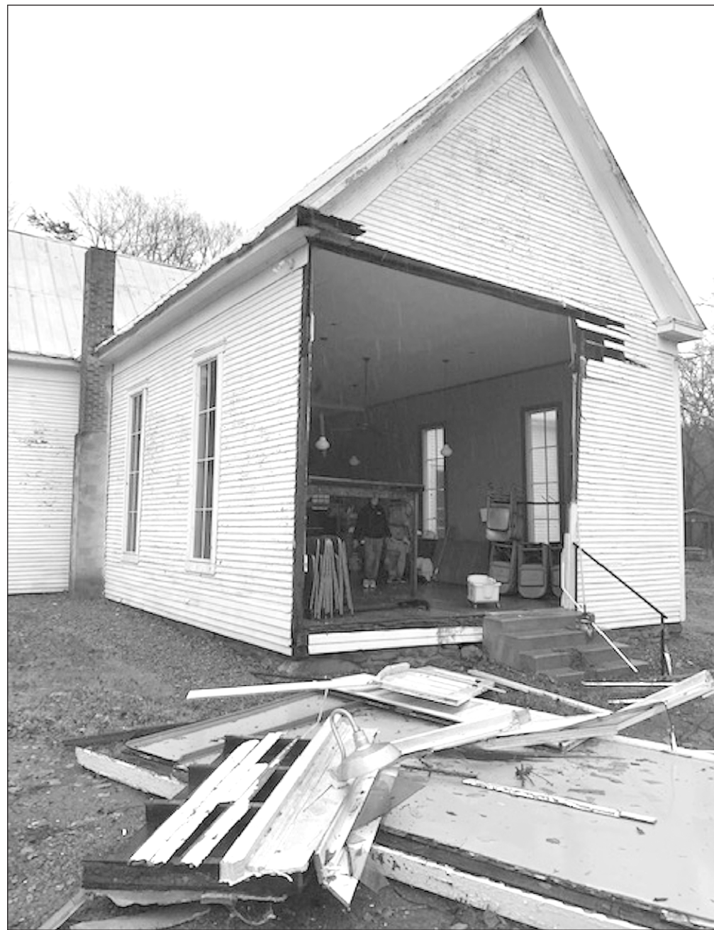
TOP: Current flooring work is underway at Raus Schoolhouse.
