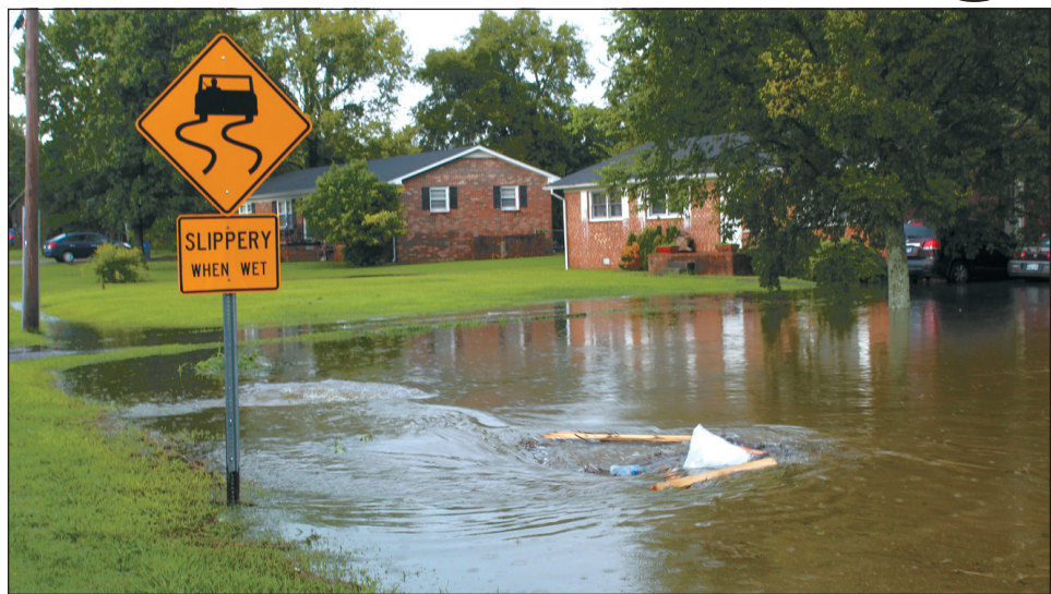
Water boils up from the system next to the Anderson home that controls water during normal conditions.
