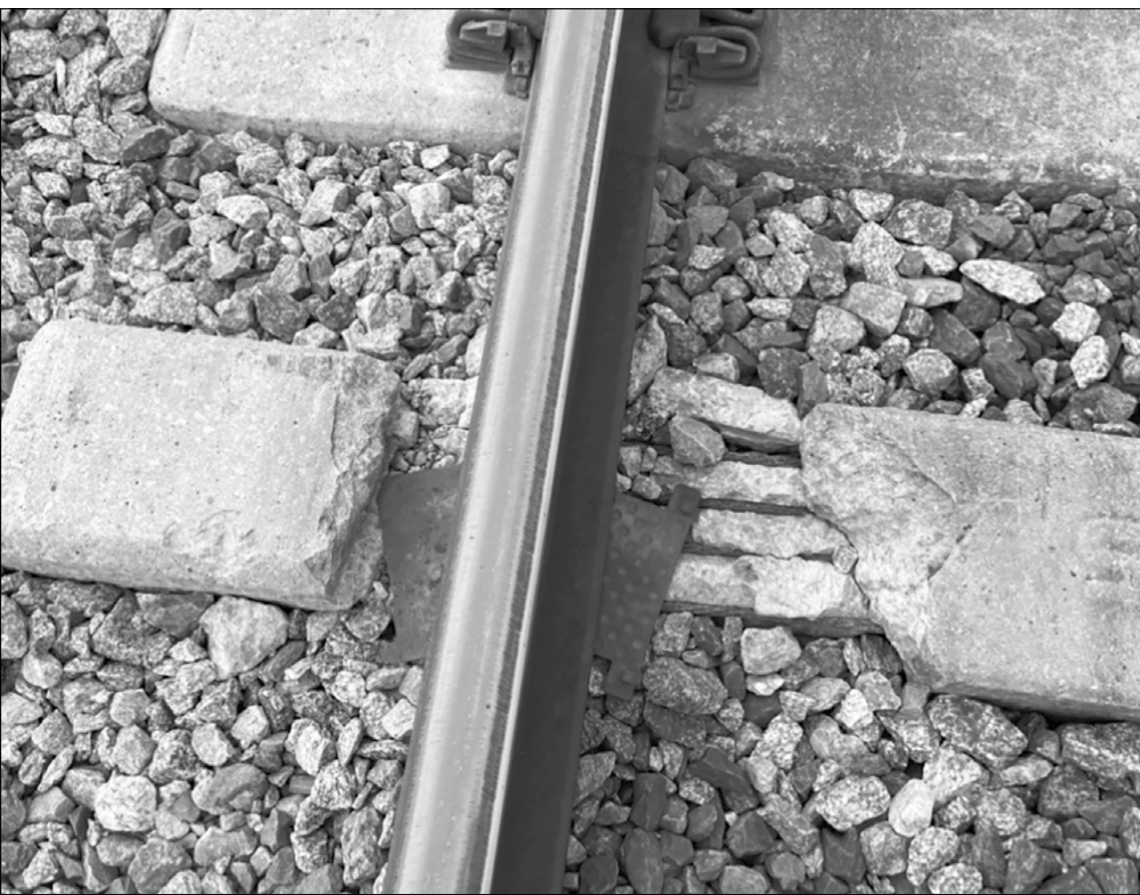
Submitted photo Due to the Ohio train derailment, Bell Buckle resident John Anderson said he is helping to form a Bell Buckle town safety committee to update their evacuation plan. This began when he noticed that one of the lines running through Bell Buckle has a crushed concrete tie. He said the spot of concern is about 30 yards to the north of the railroad and highway 82 intersection.
