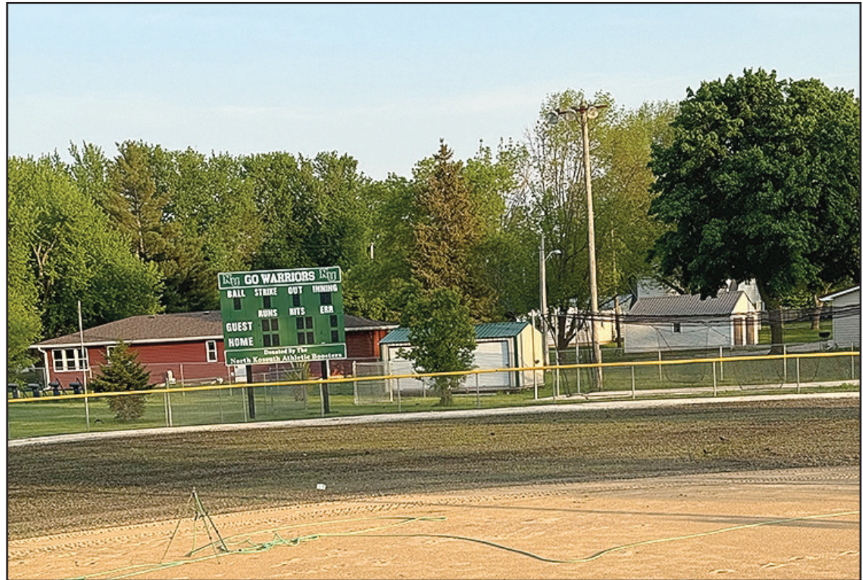
The North Union High School softball team was receiving a facelift on Monday, May 13th and Tuesday, May 14th. The grass in the outfield was removed and the dirt was prepared in order for new sod to be laid down. Due to the overly wet spring, the work was delayed and games cannot be played on the field for a few weeks. The first few softball games of the year will be played at the softball diamond in Bancroft, which is located to the south of the Bancroft Memorial baseball field.
