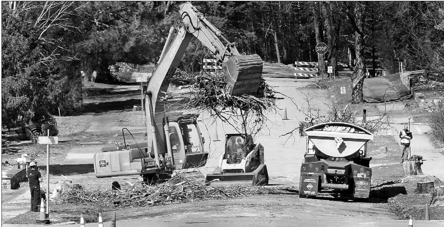
Dozens of trees lining several blocks of James Street were cleared last week by Fenske Tree Service and Mesabi Bituminous to make way for a major reconstruction project this summer. The project was scheduled to start this week with the establishment of a temporary waterline from Central Ave to Third Avenue. More information on the project can be found on the city of Ely website at www.ely.mn.us - 2020 James Street Project. photo by K. Vandervort
