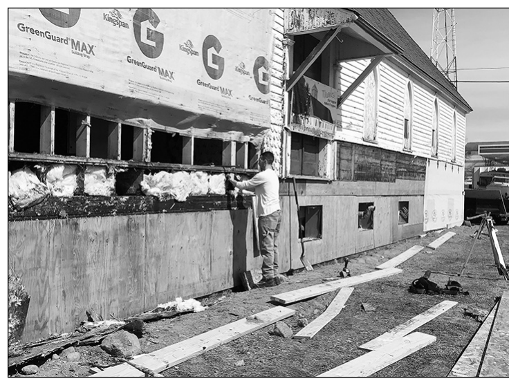
Contractors removed the old siding, installed new basement windows, did repairs and insulating, and then the new siding was ready to go up. The west side and north side siding should be ready to go up this summer.
