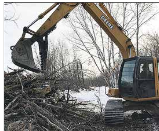
A backhoe operator was on the site of the Rose RV park last week. Tree clearing and road work is underway. photo by M. HelMBERGER
