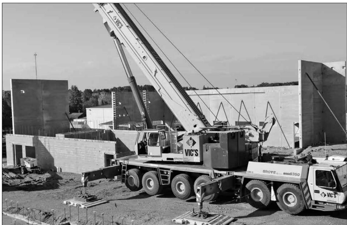
Placement of the precast walls has been the recent focus of construction crews at the Ely school building project. A 350-ton crane was used to lift the panels off of as many as 10 semi-trailers each day. Steel roof joists are stacked nearby to install by the end of the month. Warm temperatures and dry weather have made for favorable building conditions as crews hope to work indoors once winter arrives. photos by K. Vandervort
