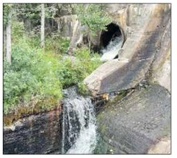
Dam's former penstock, which once held the dam's turbine, continues to leak water, contributing to the drop of the water level in the Pike River Flowage. The penstock has leaked for years, but the ongoing drought has made the extra leakage a bigger problem than
