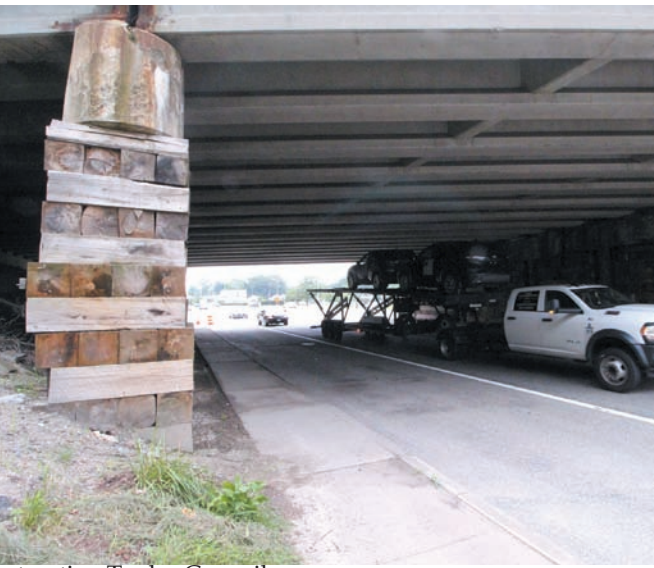
IT’S GOING TO COME DOWN: The Route 37 ramp over Post Road, now supported by wooden “logs” that looked to be swayed under the load, will come down and replaced by an at-grade intersection. Above, Derek Torrey from the Federal Highway Administration addresses the July 21 press conference at Balise Auto to announce a federal $25 million grant enabling the project. ( Warwick Beacon photos )
