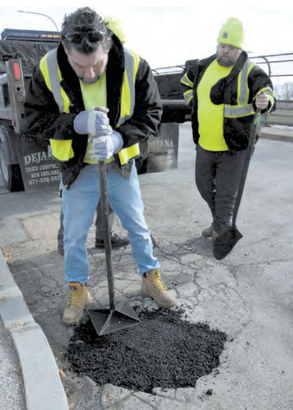
It's not going to hold unless you tamp it down good. Rocco Celletti, tamps down the patch, which could last a matter of months -- depending on the weather. (Beacon Media photo by Barbara Polichetti)
